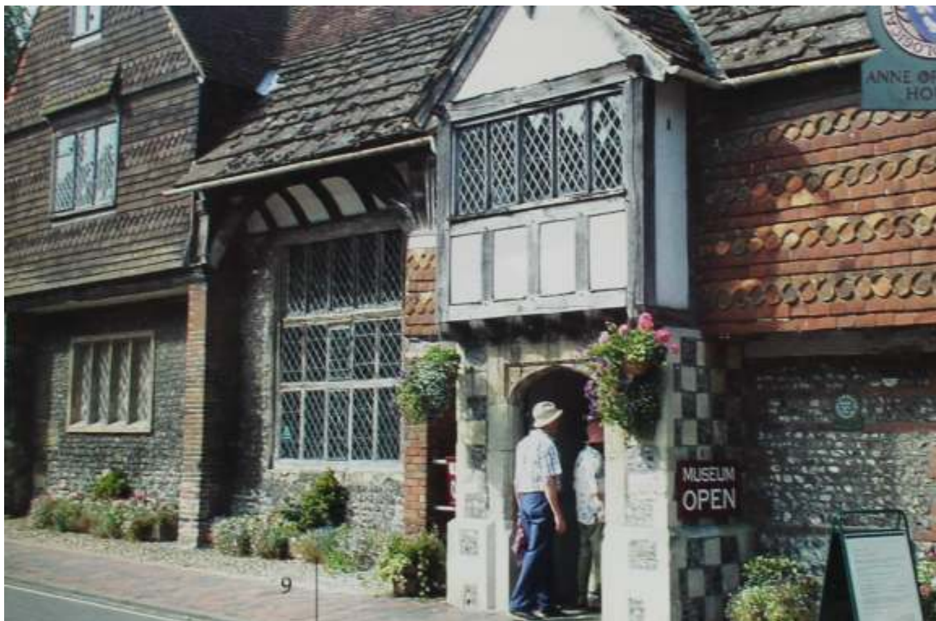
Anne of Cleves House (with acknowledgement to Lewes Town and District Councils)
